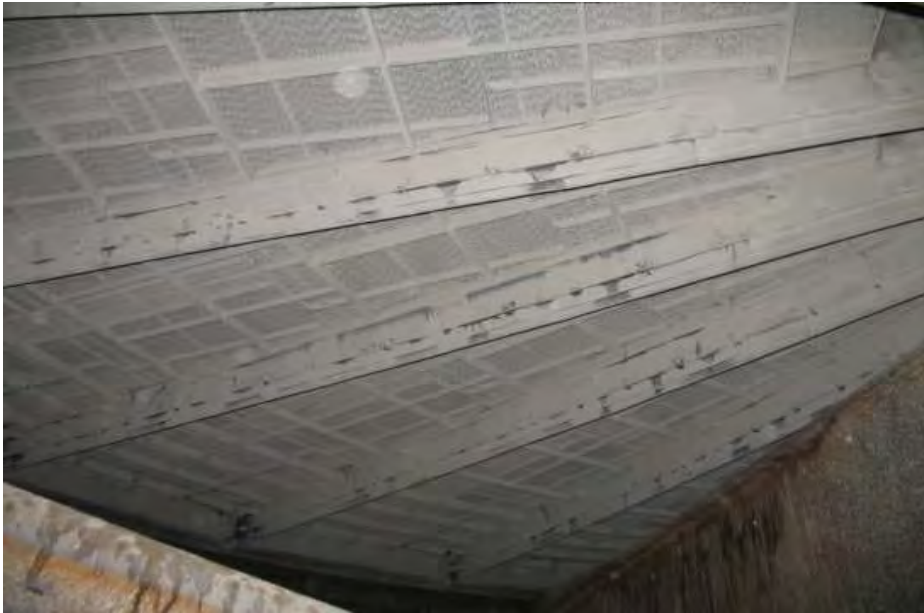
Cold-end baskets with 15 years operation
